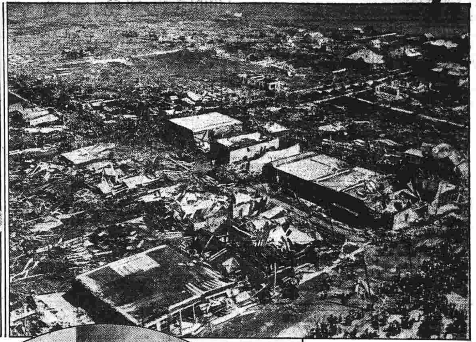
WHAT WIND CAN DO. HOUSES AND STORES, SCATTERED LIKE A BOX OF MATCHES IN A TEXAS TOWN, BY A TORNADO.
